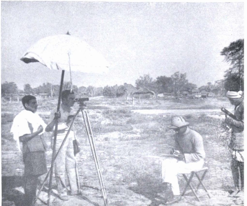
Bottom. —Secondary leveller at work on the Kosi Project survey.
